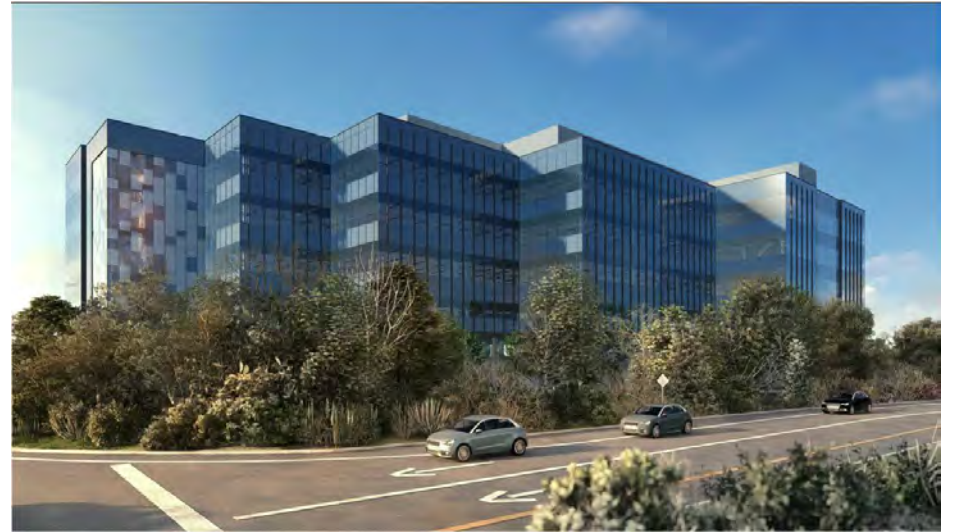
View Looking West from Holly Street / SB 101 Offramp Intersection
