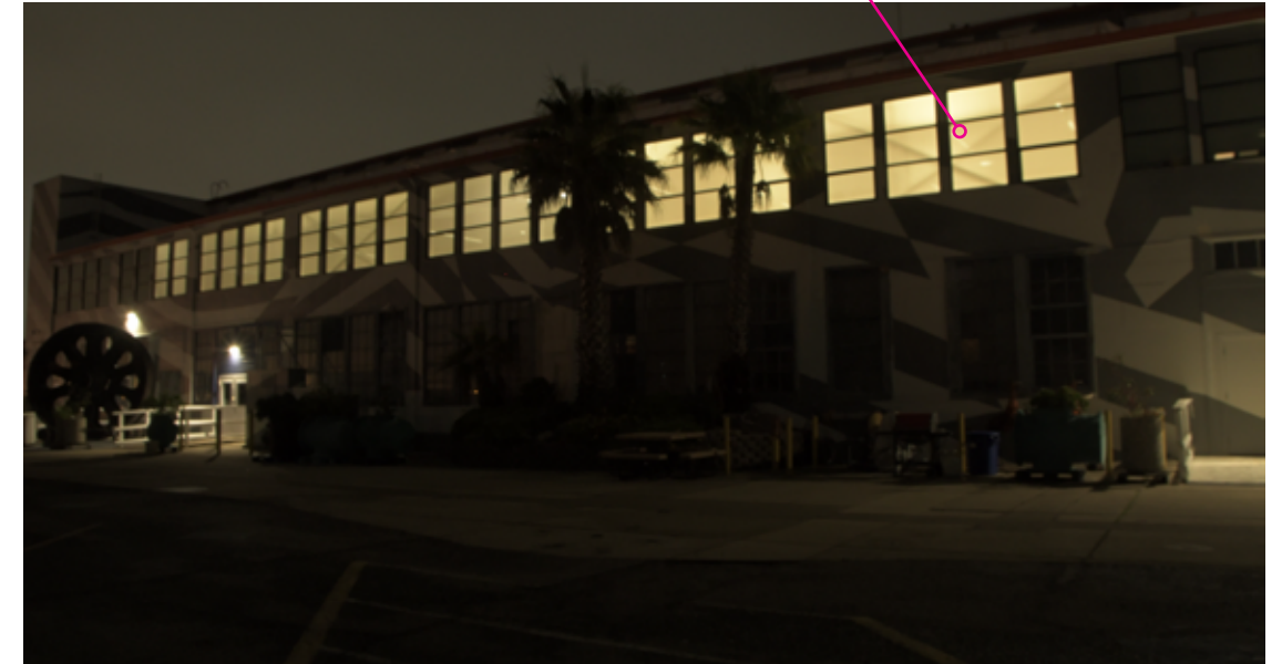
Roller Shades Deployed
