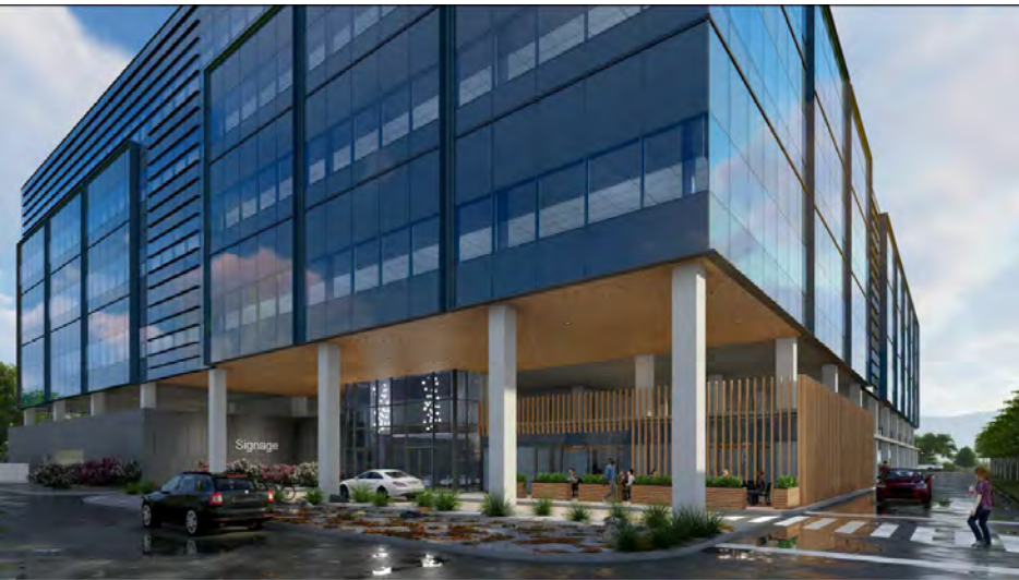
View of Main Entrance (Building's Northwest Corner)
